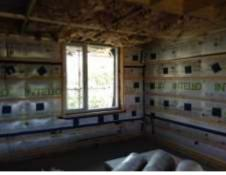
This is a high performance thermal insulation for timber framed houses. The thickness of the insulation is 300mm and it is usually blown into the spaces through holes in the internal vapour control layer. The tight packing of warmcel means there are less gaps for heat to escape in winter or warmth to come in summer. External breathable layers reduce the risk of condensation and mould growth. Our experience is that the structure loses little heat in the winter and keeps cool in the summer.
