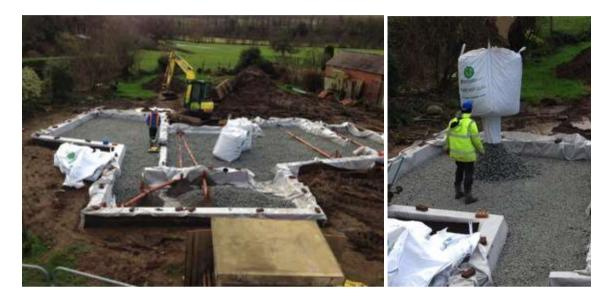
This is commonly used in retrofit buildings. It has good structural ability, drainage, is inert, fire resistant, odourless, no capillary action (prevents soil moisture coming into the building), frost proof and easy to handle.
